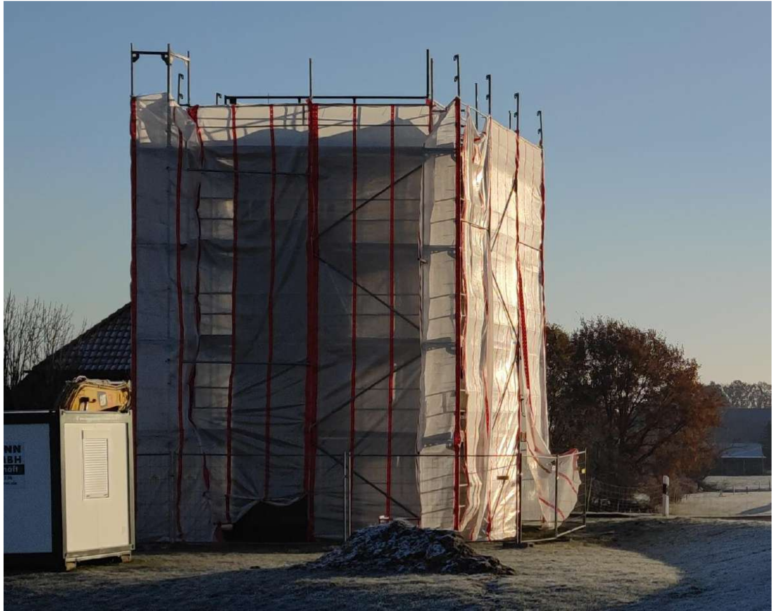
Restoration of a border tower from the time of the German division East West
