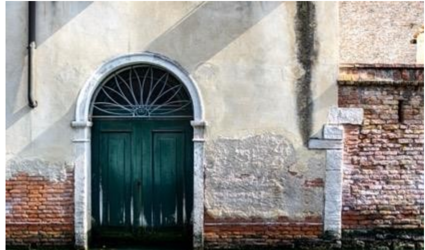
Water and salts destroy the masonry
