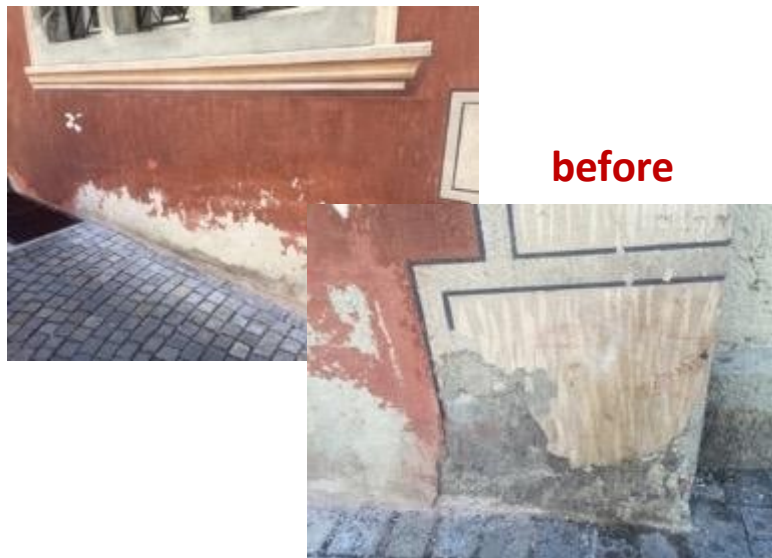
Salt-damaged outer plinth
