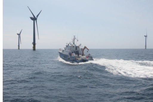
Offshore Wind Energy
